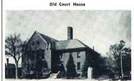
Original Cherry County Courthouse. The original home of the Valentine Public Library
